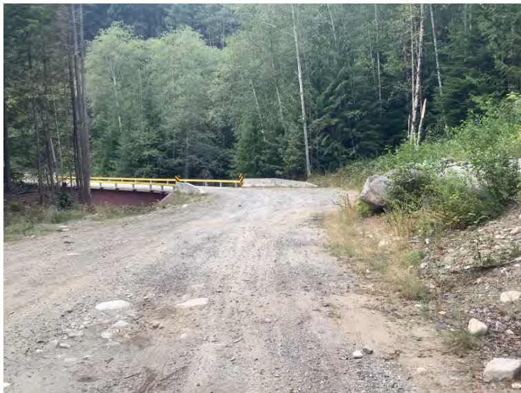
Left Bank Abutment when facing downstream
