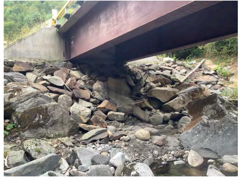
Right Bank Abutment when facing downstream
