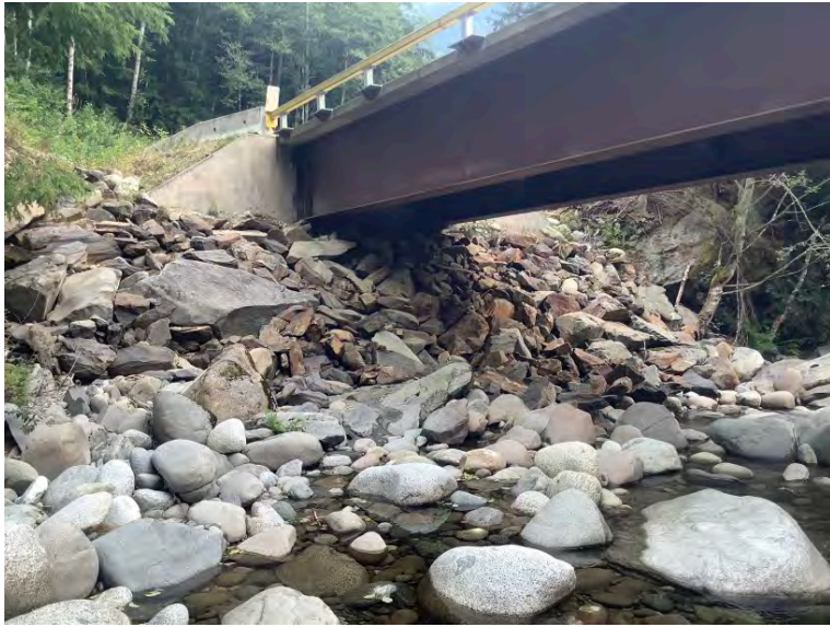
Left Bank Abutment when facing downstream
